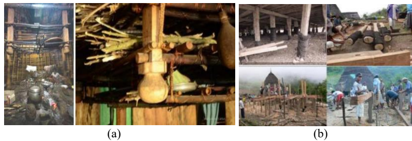
Figure 9. (a) The kitchen is placed inside the Mbaru Niang; (b) Mbaru Niang Foundation (Source: Roosandriantini, 2019)
