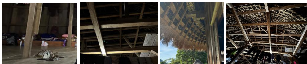
Figure 8. Illustration of Knock-down Construction on Mbaru Niang (Source: Photo by Edward V. Gunawan (2025), used with permission)
